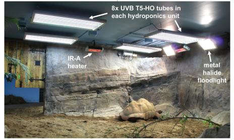
**Figure 4:** A group of four 8-tube hydroponics fixtures holding 12% UVB tubes, combined with patio IR-A heaters and metal halide floodlights, used to create a 'patch of sunlight' with UV Index 3–4 across an area 5m wide, for a group of Aldabra giant tortoises at Paignton Zoo, UK.
