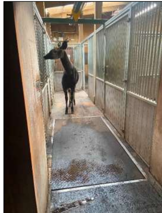
Figure 42 – Rubber mats covering the floor of a transfer lane between two stables. ©Chester Zoo / Location: Chester Zoo
