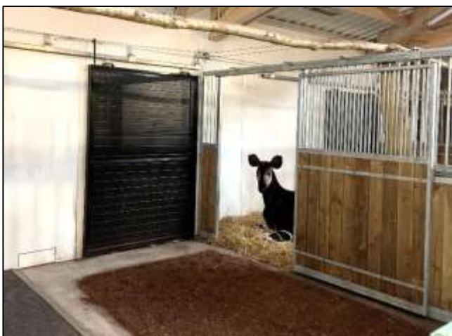
Figure 32 – Sliding doors that allow the combination/separation of multiple stables. ©Branféré Zoo / Location: Branféré Zoo
