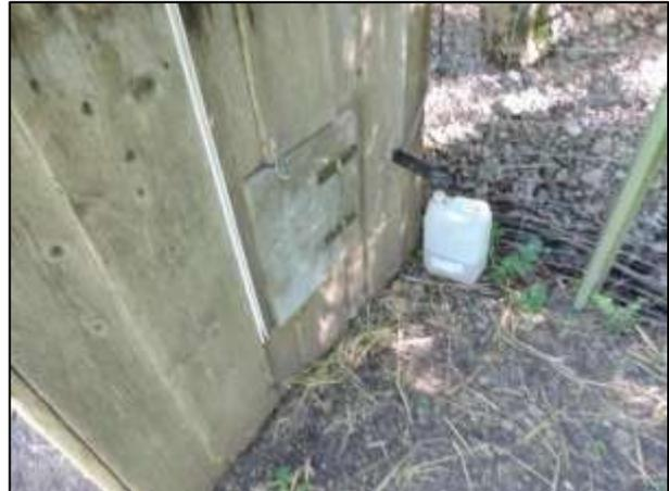
*Figure 91 There is a construction to give water through a pipe from the outside, without disturbing the chick*
