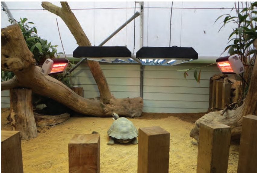
LEFT: TWO QUARTZ-HALOGEN HEATERS AND TWO UNITS OF SIX UV-B FLUORESCENT TUBES PROVIDE A LARGE BASKING AREA FOR TORTOISES IN A NATURALLY-LIT ENCLOSURE. RIGHT: MONITORING THERMOREGULATING TORTOISES IN REAL-TIME USING A THERMAL-IMAGING CAMERA
