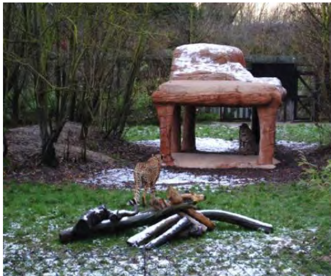
Figure 6: Shelter with floor (and roof) heating (Colchester Zoo)
