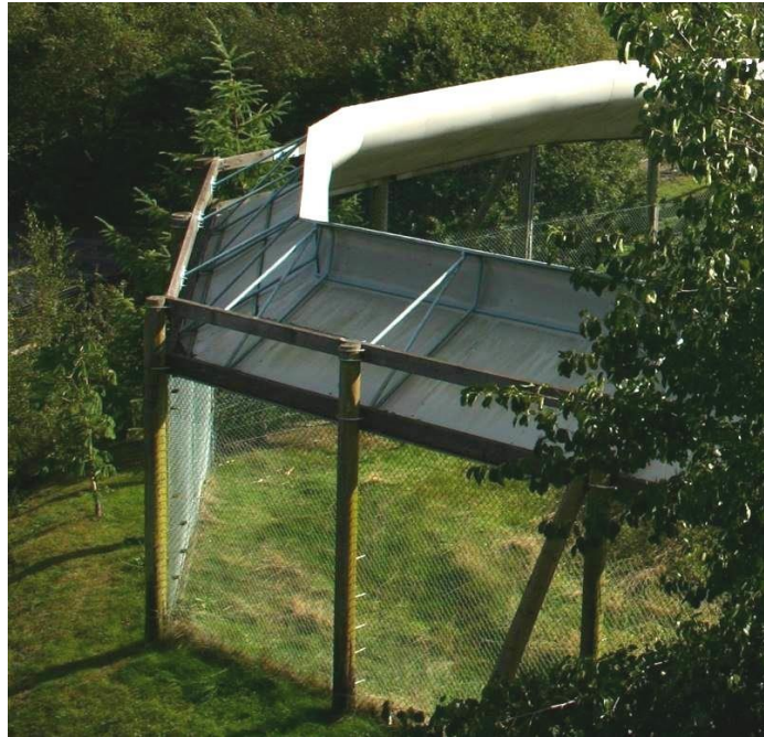
Fig. 10. Smooth overhanging structure as containment on top of a chainlink fence in Monkeyworld (Wareham). Note the hotwires to protect both the lower and upper sections of chainlink.
