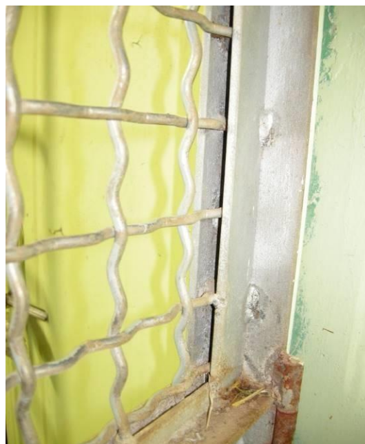
Fig. 8 Wave mesh welded between steel profiles.
