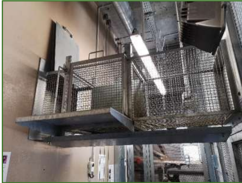
Figure 21 - Passage with crush tunnel system for catching sifakas at Paris Zoo. © Björn Unger
