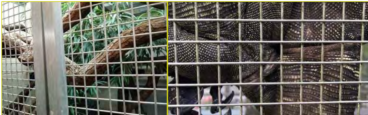
Figure 27. (Left) One-inch square stainless-steel mesh, used to construct off-show crocodile monitor enclosures at Marwell Zoo. Photo: Rob Haines, Marwell Wildlife. Figure 28. (Right) Detail of stainless-steel mesh used at the Singapore Zoo. Photo: Borja Reh
