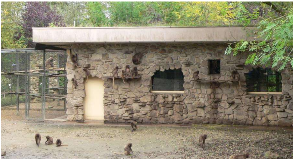
Fig 57 The wall of the house allows the geladas climbing exercise. Shelves are preferred places for resting and sleeping. Note the windows which allow the animals to look out when indoors (and in when outdoors) / NaturZoo Rheine
