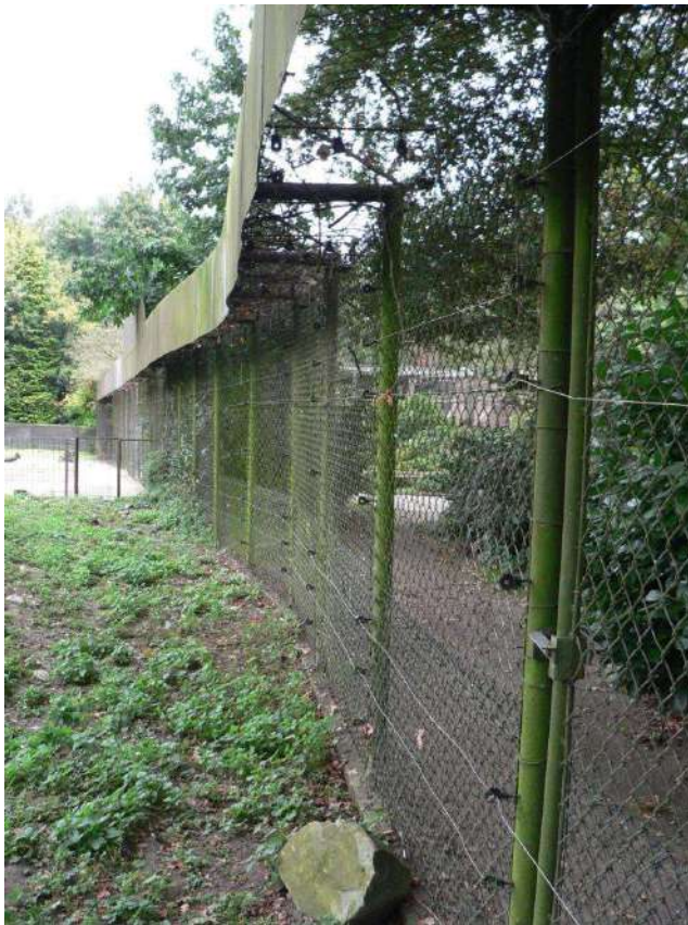
Fig 26 Fence with overhanging structure / NaturZoo Rheine
