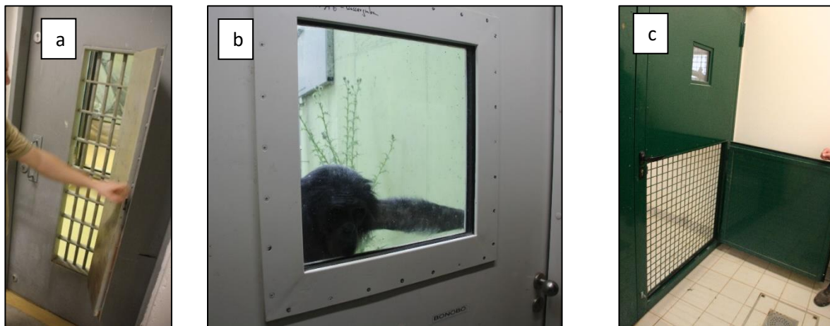
Figure 16: Examples of "double doors" where visibility is guaranteed, but noise levels can be reduced (a: Leipzig Zoo – Jeroen Stevens; b: Frankfurt Zoo – Jeroen Stevens, c: La Vallée des Singes – Jeroen Stevens).
