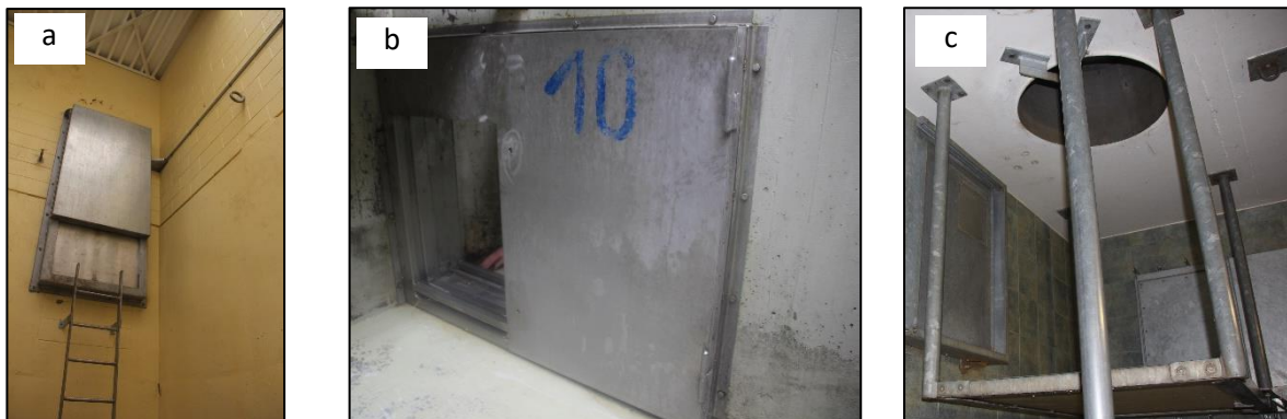
Figure 24: Different sliding doors in bonobo exhibits. a: door that slides in a vertical plane (guillotine door) (Milwaukee Zoo - Jeroen Stevens); b: door sliding in a horizontal plane (Cologne Zoo - Jeroen Stevens); c: sliding door in the ceiling connecting enclosures that are on top of each other (Leipzig Zoo – Jeroen Stevens).
