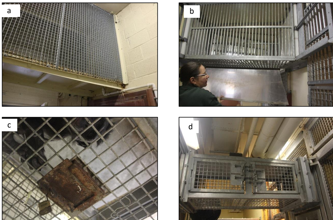
Figure 28: Designs for overhead tunnels in bonobos. a: Solid bottom tunnel with water drainage (Planckendaal – Jeroen Stevens); b: Wire bottom tunnel with plastic sheet protection (Apenheul – Jeroen Stevens); c: Small door in tunnel bottom for ultrasound inspections (Milwaukee Zoo – Jeroen Stevens); d) Side doors to be able to remove sedated bonobos from the tunnel (Milwaukee Zoo – Jeroen Stevens).
