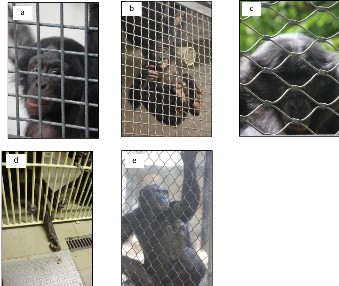
Figure 23: Types of mesh used for bonobo enclosures. a: Welded mesh (La Vallée des Singes – Jeroen Stevens); b: Wave mesh (Cincinnati Zoo – Jeroen Stevens); c: Woven mesh with metal clips (Cologne Zoo – Jeroen Stevens); d: Steel bars NOT RECOMMENDED- showing how individuals can reach through (Planckendael – Jeroen Stevens); e: Chain-link mesh – NOT RECOMMENDED (Milwaukee Zoo – Jeroen Stevens).
