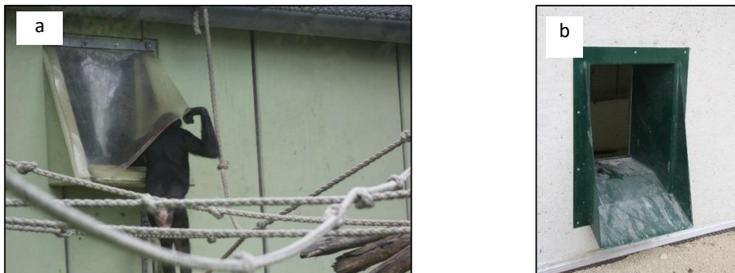
Figure 27: Designs for doors between indoor and outdoor enclosures. a: plastic sheet to prevent draught with system to close relatively tight (Frankfurt Zoo – Jeroen Stevens); b: Slightly angled tunnel to prevent dirt accumulating in the tunnel (La Vallée des Singes – Jeroen Stevens).
