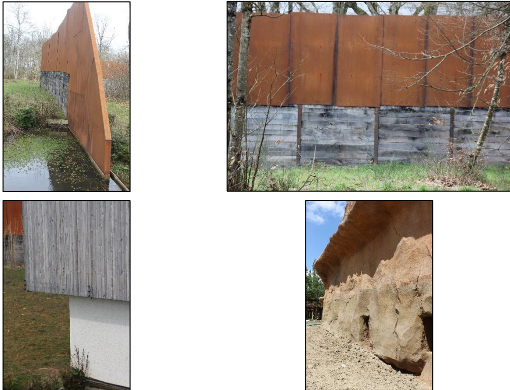
Figure 19; Examples of designs for enclosure walls that have proven to be effective a-b: Wall covered with metal sheet, note that in front of the base of the wall electric fences and planting have been used (La Vallée des Singes - Jeroen Stevens); c: overhang, with additional electric fence as secondary barrier (La Vallée des Singes – Jeroen Stevens); d: rockwork wall with overhang (Zoo Planckendael – Jeroen Stevens).
