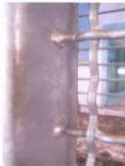
Mesh welding to frame (terminal)
